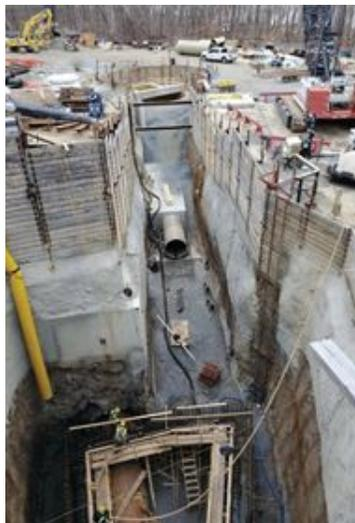
Flow fill installation to block identified sewage leak between SOE walls of new & existing MH31
