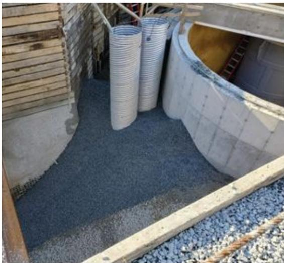
Stone backfill & dewatering corrugated metal sumps to pump sewage identified leak between SOE walls of new MH31 and existing MH31
