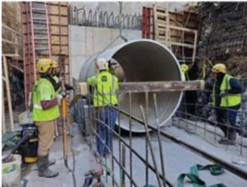
Installation of new 78" HOBAS pipe between new MH31 and new MH30.59
