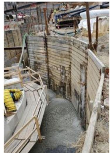
Installation of 78" HOBAS pipe & concrete encasement
