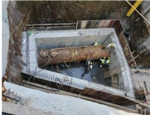
Installation of concrete walls at new MH30.59
