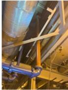
PSW Nitrogen Pipe removal and installation of a new one.
