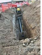
East & West Primary Sludge Replacement Pipes Installation
