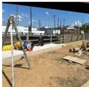
Backfilling trench & concrete slabs for cabinet support.
