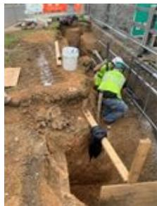
Excavation and installation of rebar for concrete slabs for DC Water I&C and PEPCO cabinets.
