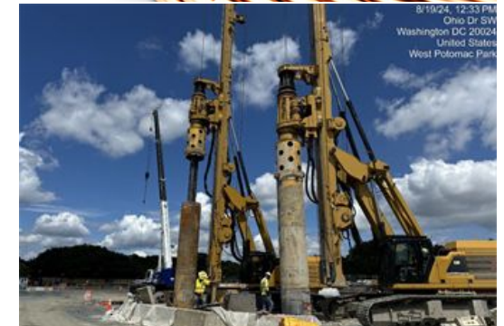
DCCR Potomac Tunnel Mining Shaft Construction
