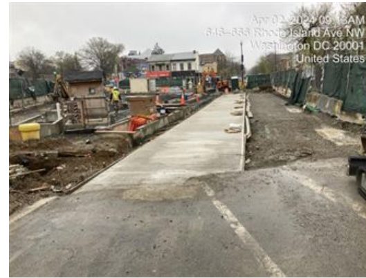
R Street - Site Restoration
