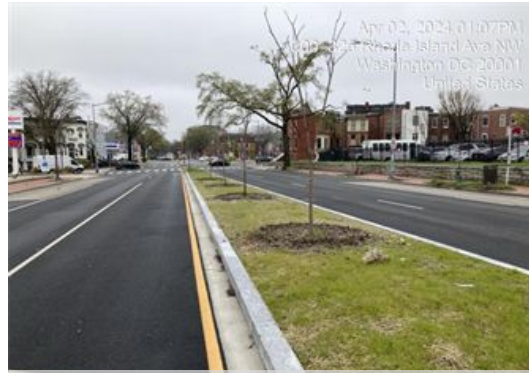
Rhode Island Avenue - Median Restoration & Landscaping
