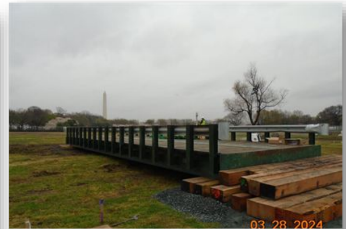
Temporary Bridge Over Force Mains
