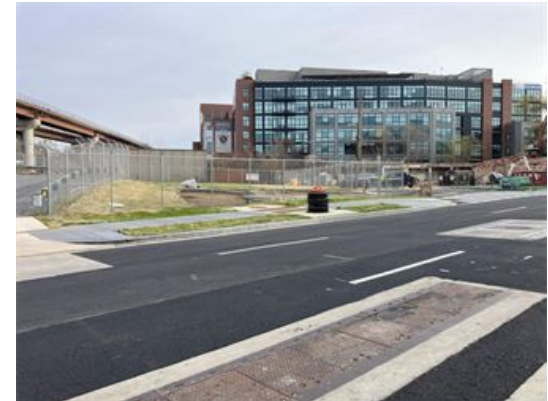
Rhode Island Avenue - Site Restoration
