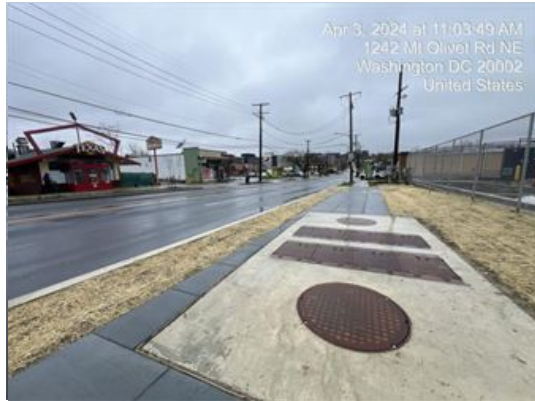
MOR - Site Restoration
