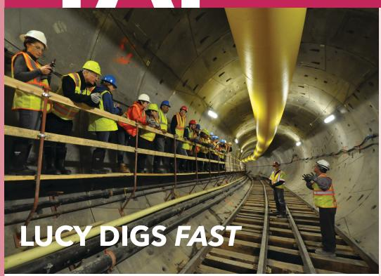
DC Water's third giant tunnel boring machine (TBM), named Lucy, finished her tunnel segment, completing a 2,700 foot long, 20.5-foot diameter tunnel called the First Street Tunnel. She mined under First Street, NW (about 100 feet underground) from Channing Street to Rhode Island Avenue, and had to cut her way through 500 million pounds of sand, silt and clay.
