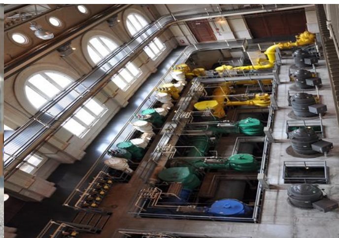
Bryant Street Pump Station
