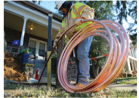
Replacing lead service lines with copper pipe is an important step in reducing lead risk
