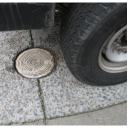
the meter is read remotely by the use of radio frequency and satellite technology. Two readings a day are uploaded to DC Water.
