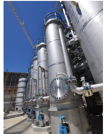
CAMBI thermal hydrolysis vessels – a first in North America
