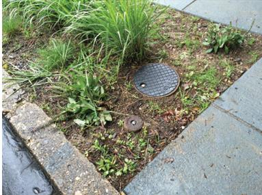
When DC Water needs to access the meter pit, for meter replacements, valve shut offs, or other emergencies, crews do their best to limit disturbances to landscaping. They try to gain entry to the meter pits on the side closest to a driveway or sidewalk. This amount of space to access the meter pit should always remain clear. This is the best way to avoid estimated bills and to ensure accurate and timely billing.
