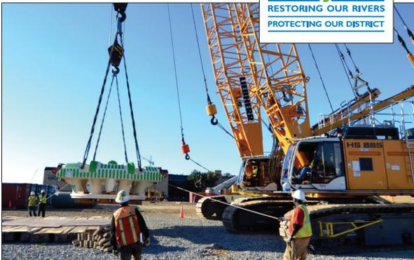
The Tunnel Boring Machine (TBM) arrives on Blue Plains. It is slated to begin boring the first tunnel in early 2013.
