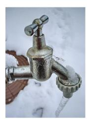
Extreme cold weather and freezing temperatures can damage household water pipes. Some pipes are at a greater risk of freezing depending on where they are located in the home. Unexposed pipes are more likely to freeze or burst because of a lack of insulation and heat.
