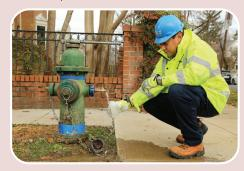
Further, sometimes hydrants are opened to blow off excess water so repairs can be made to a valve. The water pipe has to be empty in order for the repair to happen, so excess water is diverted away, usually into the street and down the storm drain.
