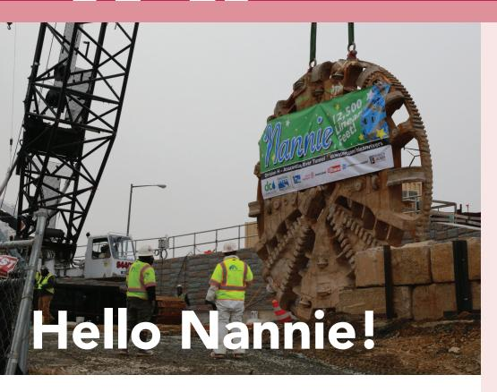
Starting the year off with a victory, DC Water and its contractor, Salini-Impregilo / Healy / Parsons (IHP) joint venture, lifted the face of the latest massive tunnel boring machine (TBM), Nannie, from a depth of 102 feet to the surface.
