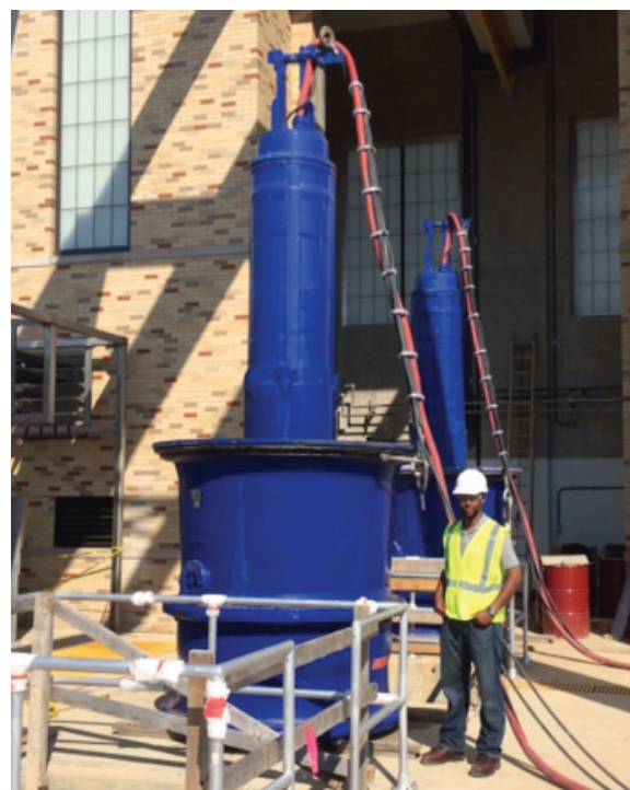
The new pumping station includes these 450 hp pumps
