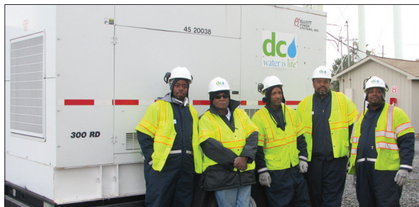
Five DC Water employees delivered a 300-kilowatt generator to Long Beach Township, New Jersey, to assist in bringing that community's wastewater system back online after Tropical Storm Sandy.
