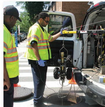
DC WASA crew lowers robotic camera into manhole to perform sewer investigations.
