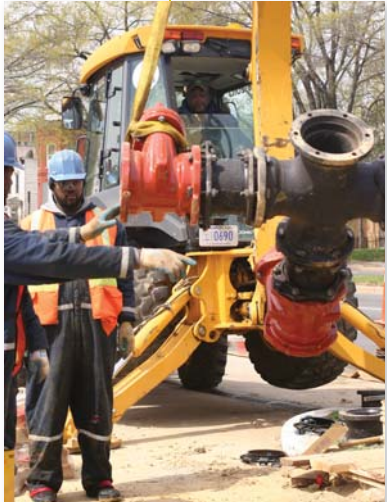
WASA is replacing old, inoperable valves throughout the District.
