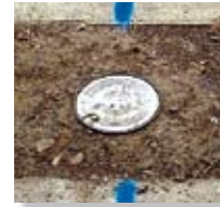
A painted line (in the above photo, blue) marks an underground utility.
