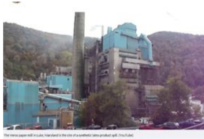
The Verso paper mill in Luke, Maryland is the site of a synthetic latex product spill. (YouTube)
