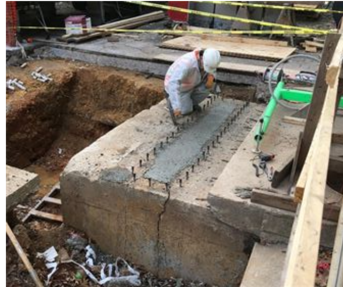
Repairs to Stop Log Chamber
