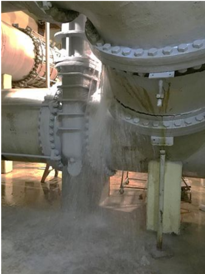
Piping segment leaking at failed flange
