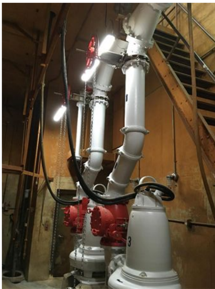
New Pumps and Piping Installed
