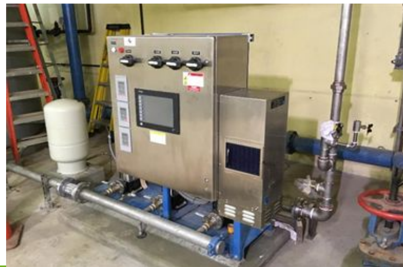
New Seal Water Pump Skid and Controls
