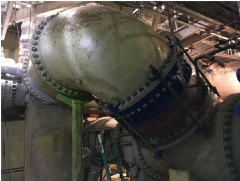
Repaired piping segment
