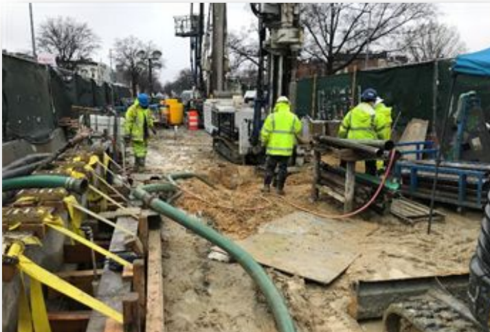
Adit/Tunnel Connection Ground Improvement
