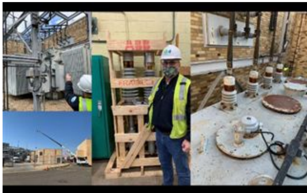
Figure 1. Ray Thompson, Foreman, High Voltage Power Distribution, manages the day-to-day activities of DC Water’s High Voltage maintenance contractor, which performs preventive maintenance inspections on critical electrical systems, including the three incoming transformers.
