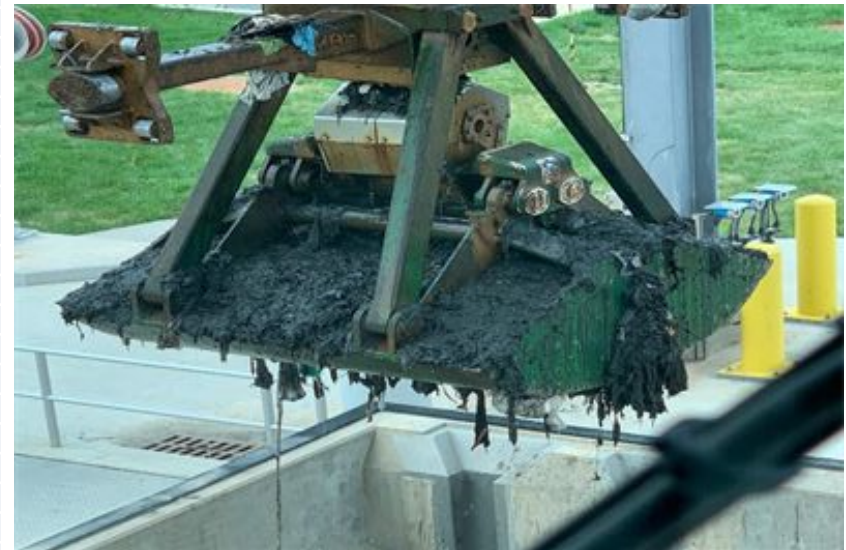
Trash, Debris and Solids Removal from Screening Shaft at Tunnel Dewatering Pumping Station
