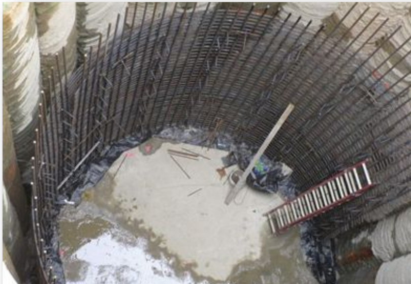
Shaft CIP Liner Rebar Installation Elev. 28.5
