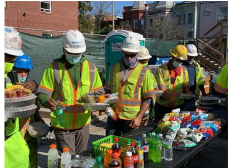
Lunch Purchase Program for Crews at T Street and Pumping Station Construction Sites
