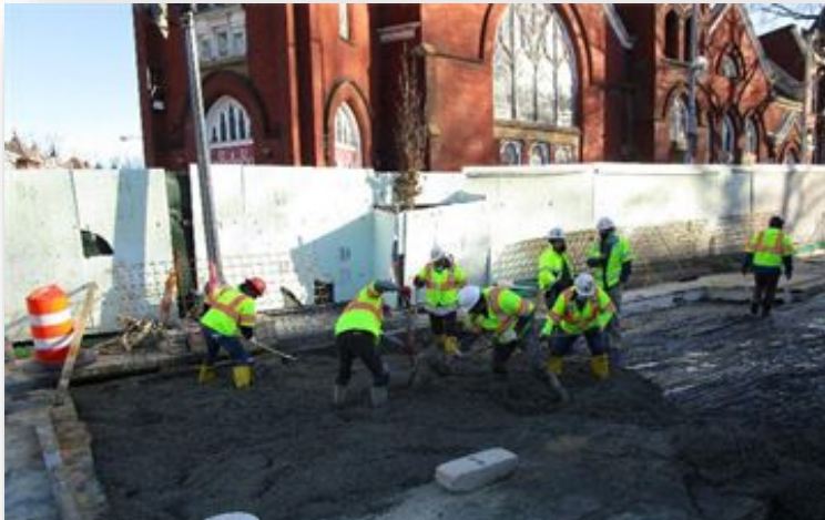
First Street Road Restoration – Pouring Concrete Base
