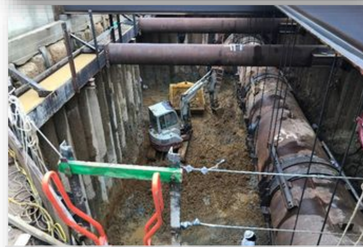
Diversion Structure Construction
