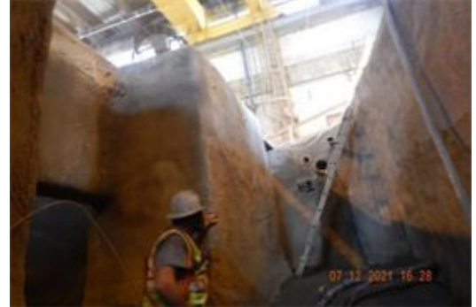
Figure 3. Restored section with calcium aluminate shotcrete
