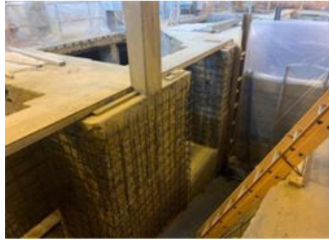
Figure 2. Installation of additional rebar
