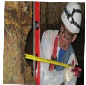
Figure 1. Up to six inches of concrete were found to be missing from existing walls with
