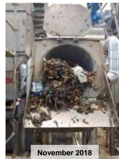
Trash and Debris Removed from CSO Captured by Tunnel at ECF Fine Screens
