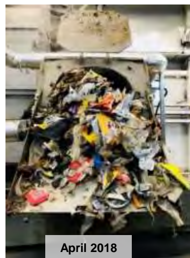
Trash and Debris Removed from CSO Captured by Tunnel at ECF Fine Screens
