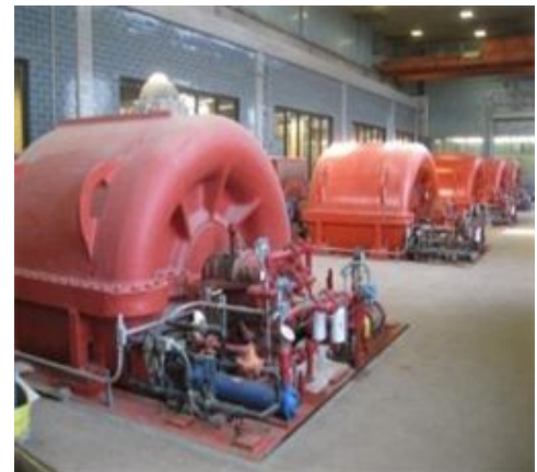
Nitrification and Effluent Aeration System consist of five 4000 Horsepower (HP) blowers (each) and air distribution pipe and diffuser systems
