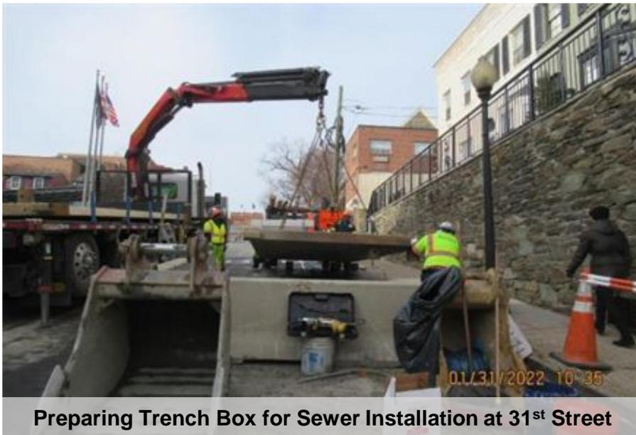
Preparing Trench Box for Sewer Installation at 31<sup>st</sup> Street
