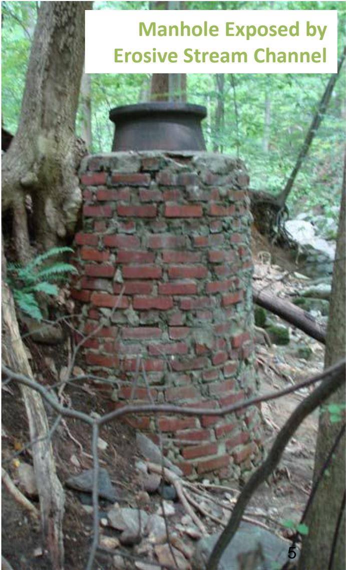
Manhole Exposed by Erosive Stream Channel
