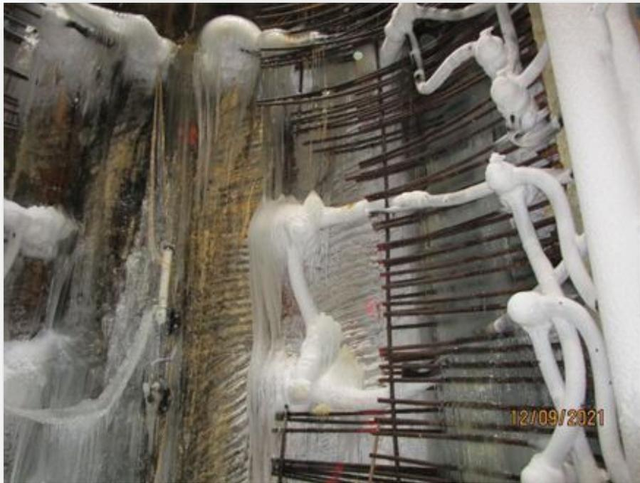
Ground Freeze System in Drop Shaft
