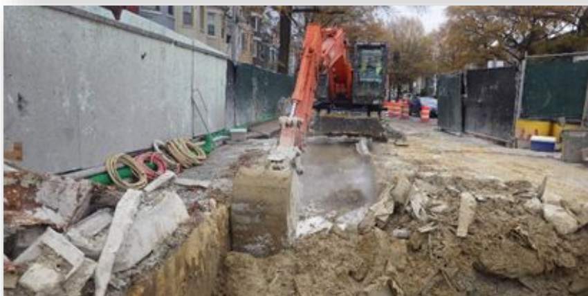
Site Restoration after Ground Improvement
