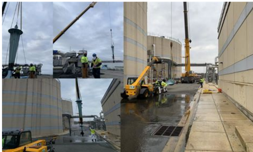
Proactive maintenance of Anaerobic Digesters mixing unit that required rigging and lifting
