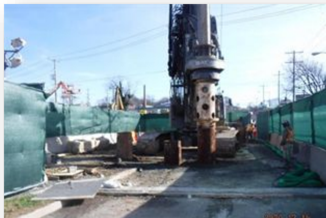
Diversion Chamber Support of Excavation
