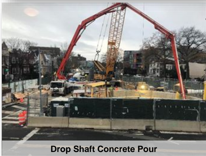
Drop Shaft Bottom Slab Placement
