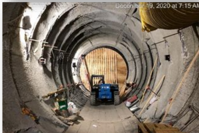
Adit Support of Excavation
