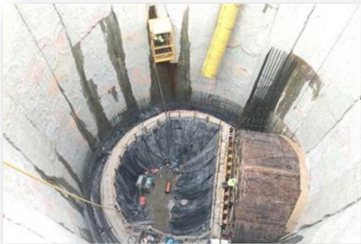
Drop Shaft Bottom Slab Placement
