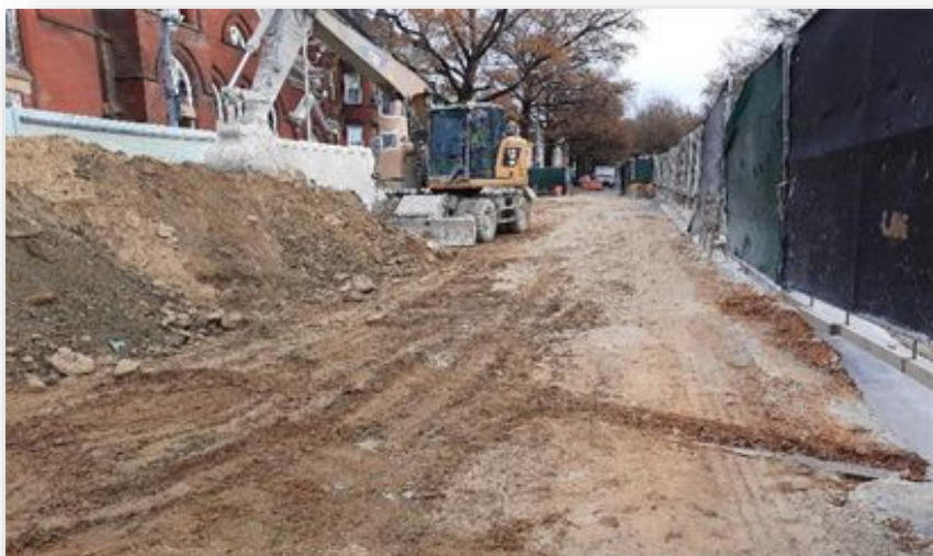
Site Restoration after Ground Improvement
