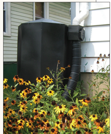
Rain barrels capture runoff from rooftops for later use around the home or garden.
