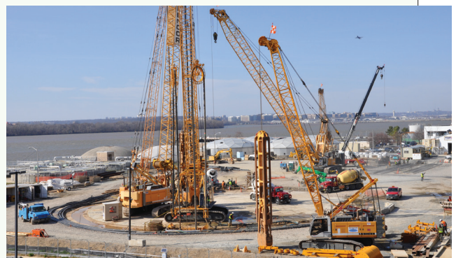
The first portion is called the Blue Plains Tunnel. Here construction begins at Blue Plains to build the shaft nearly 16 stories deep where the tunneling will begin.
