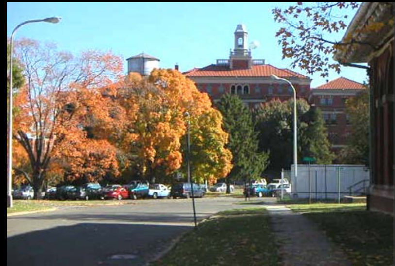
Entrance to St. Elizabeths Hospital Campus with view of existing water tower
