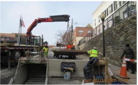
Preparing Trench Box for Sewer Installation at 31<sup>st</sup> Street
