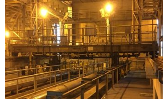
Screens, Grit & Primary Facilities Upgrades
