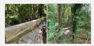
Work started to rebuild the crumbling concrete encasement around the 10-inch sanitary sewer crossing the creek at 3350 Erie Street, SE (see pictures)
