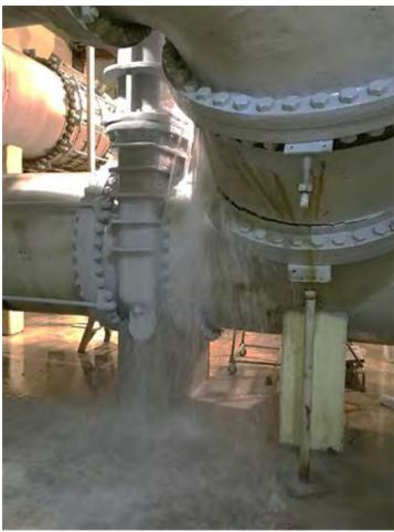
Piping segment leaking at failed flange
