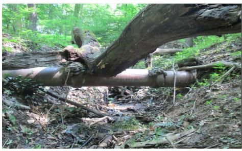
10" VCP Sewer pipe, installed in 1914, near Morrow Dr NW, located in Rock Creek Park.
