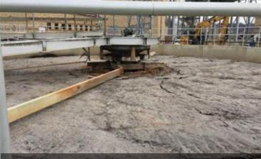
Unsettled Sludge Buildup on Surface Damaging Collector Mechanisms
