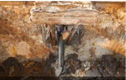
Grit Chamber I, Effluent Sluice Gate Corrosion
