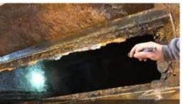
Grit Chamber Building | Concrete Corrosion
