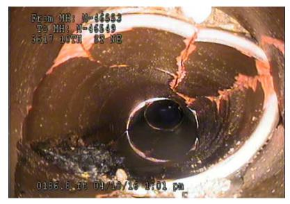
10<sup>th</sup> St at Otis St, NE (10" VCP, deformed, broken
