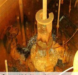
Pumps with leaking seal
