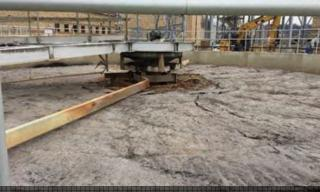
Rusted Weir Plate, Scum Baffle, and Embedded
