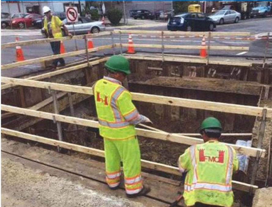
Thrust Block Installation at Rhode Island Ave & 6 th ST NW
