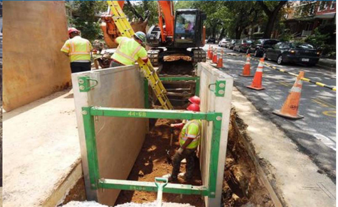
Small Diameter Water Main Replacement
