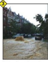
▲ Flooding at 1st and V Streets NW
