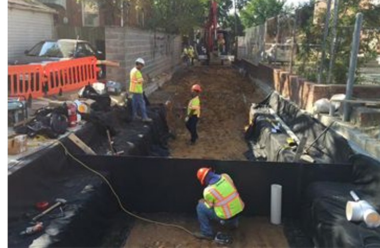
Facility ID: APP-4403
