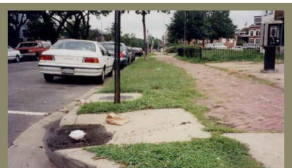
Trash on street washes into catch basin.
