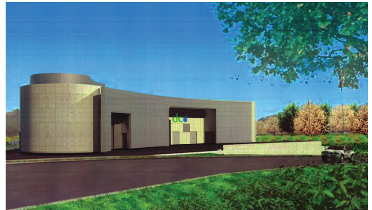
Top: Poplar Point Pumping Station – East Elevation (viewed from I-295)
