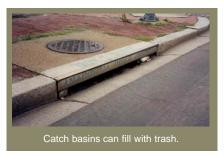
Don't use catch basins as trash receptacles or to dispose of leaves! Debris in catch basins can cause local flooding and increase the potential for dry weather overflows (see photo below).
