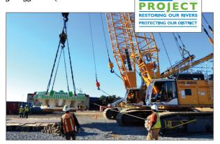
The Tunnel Boring Machine (TBM) arrives on Blue Plains. It is slated to begin boring the first tunnel in early 2013.
