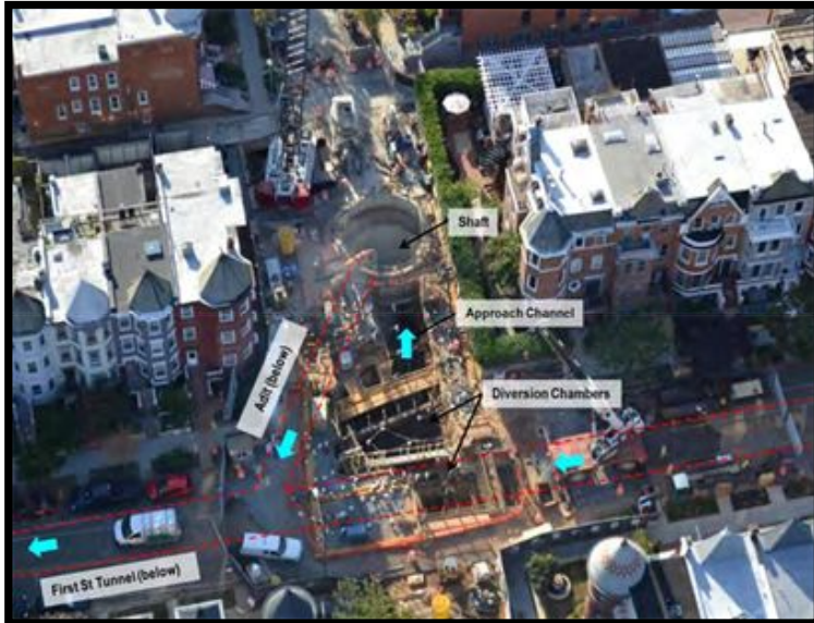
First Street Tunnel Example: First and V Streets NW, Diversion Chambers and Drop Shaft
