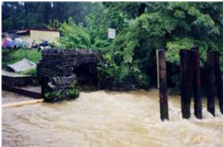
CSO Discharge to Anacostia River
