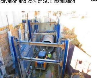
Installation of Flume Pipe for 108" Outfall Sewer
