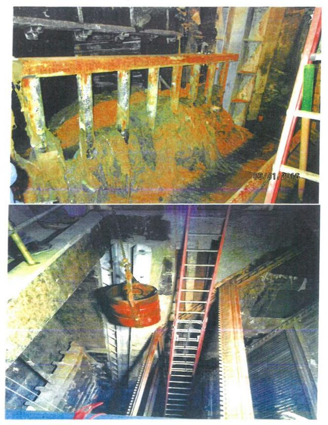
Figure 3: Wet Well Supplemental Bar Screens
