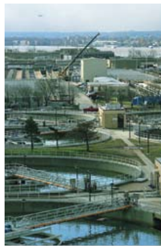
Blue Plains Advanced Wastewater Treatment Plant
