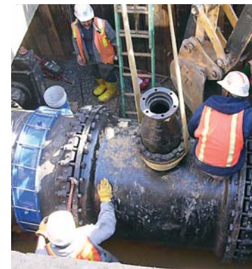
Water main improvements enhance the water distribution system.
