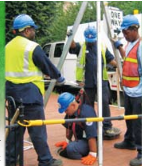
(Right) DC WASA Sewer Services crew working on Independence Avenue, SE.
