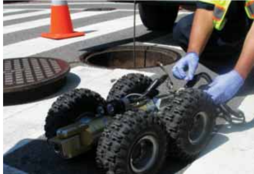
The Authority's sewer investigation team troubleshoots sewer blockages with camera-mounted, remote-controlled robots that send back live footage of sewer interiors.
