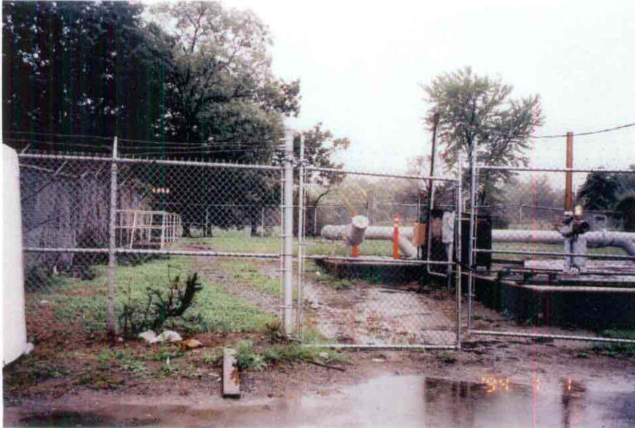
Photo 1: Existing below-grade East Side Pumping Station. View is South.
